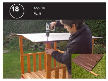
Fig. 18 Insert the crossbar (O) into the cover tarp (15). Attach it using screw (4).
